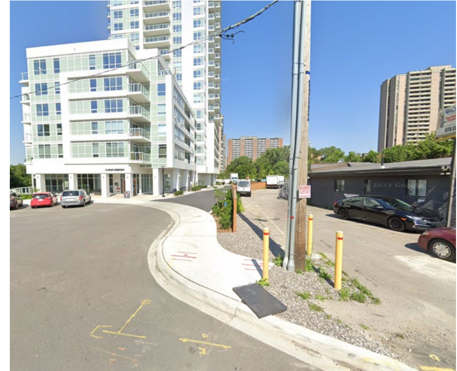
Wilby Crescent Existing Conditions (west side)
