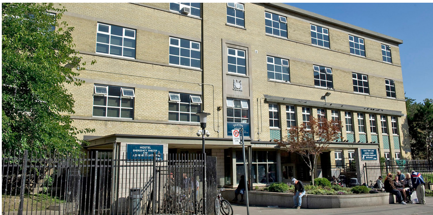
Current day Seaton House building located at 339 George St.
