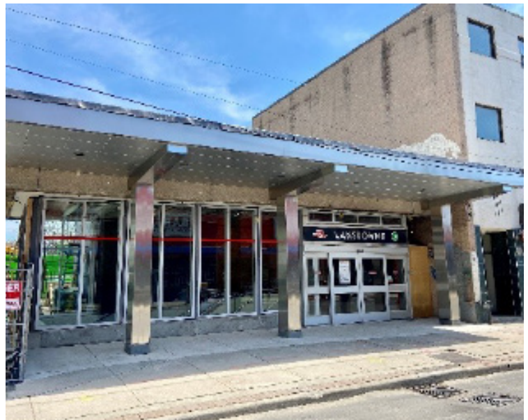
Lansdowne Station Entrance
