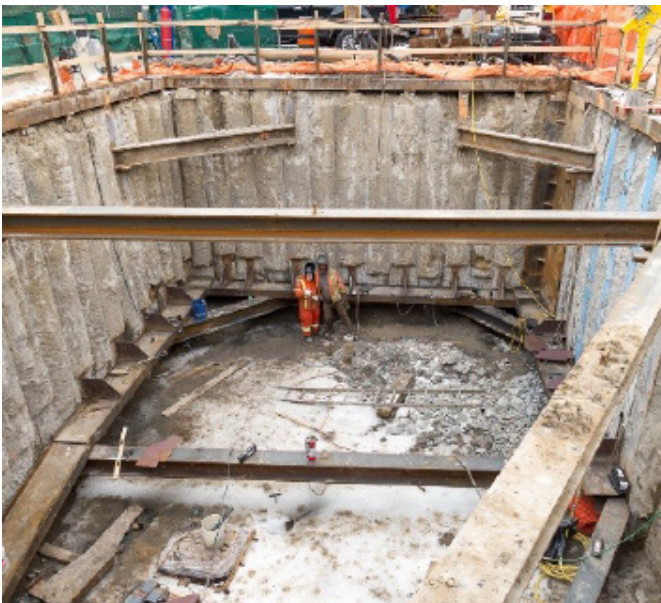
Donlands Station Excavation
