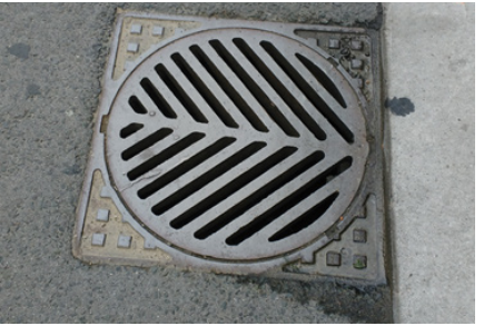
Figure 3.55 A catch basin with herring bone grates.
