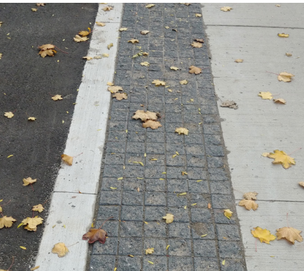
Figure 3.8 A band of visually contrasting, cane detectable unit pavers adjacent to a sidewalk elevation cycle track.
